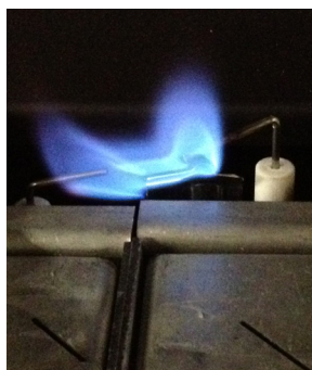
Normal Pilot Flame Pattern
