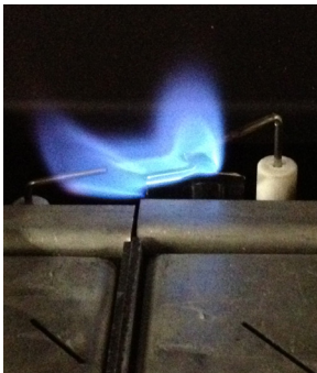
Normal Pilot Flame Pattern
