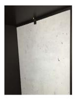
With the panel held in position, hold the slotted "L" shaped clip to the ceiling and the other end against the glass. Leave 1/16" space top allow for expansion. Use the self-tapping screw to secure the clip to the ceiling. The slot will allow you to adjust the clip.
