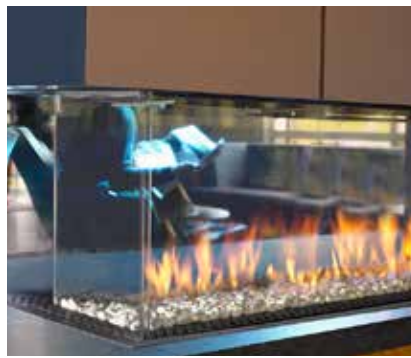
Glass Safety Barrier
