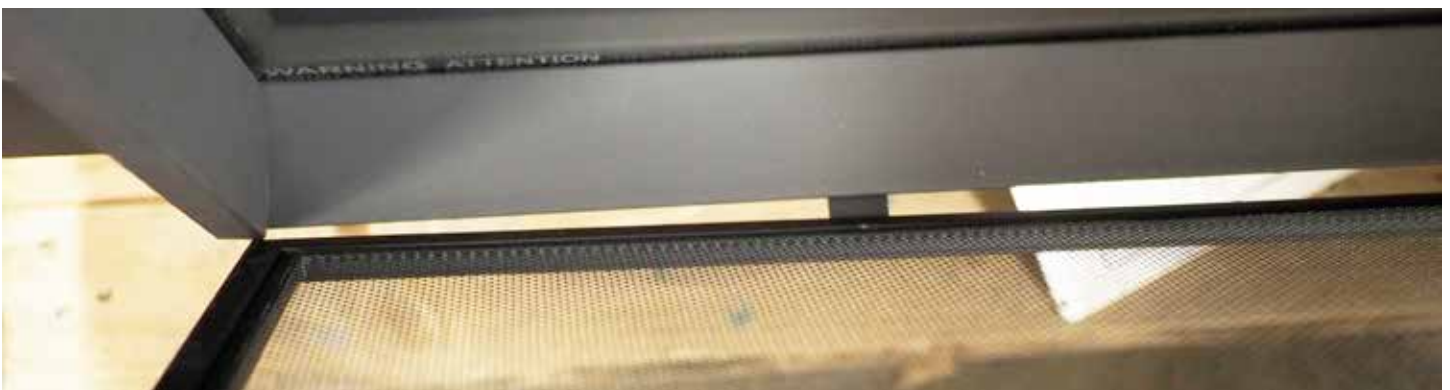
Figure 11 Rest the bottom of the screen on the 3 tabs that are under the trim. Push the screen into position so that the exposed magnets come in contact with the screen frame.
