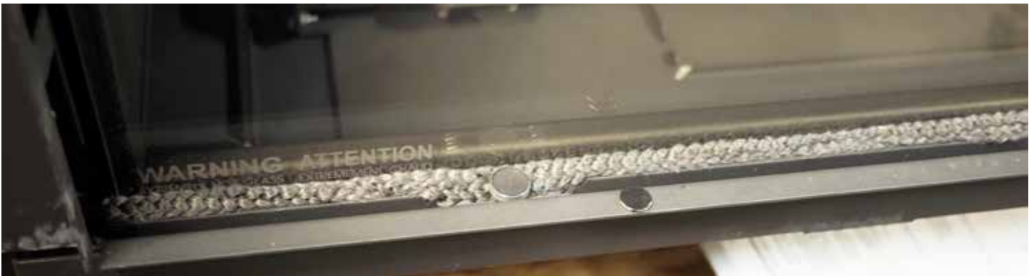
Figure 1 Place single magnet on bottom return flange 12" from the left end corner, right end corner, and the center.
