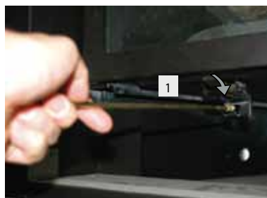
Figure 22g. Removing and installing the glass doors. (Both Sides Typical)
