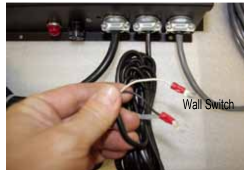
Figure 20a. Remote Switch Wire Connection
