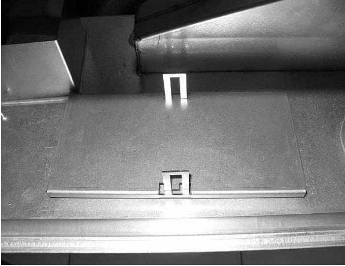
Figure 16 - Relief Door Showing Line-up Tab
