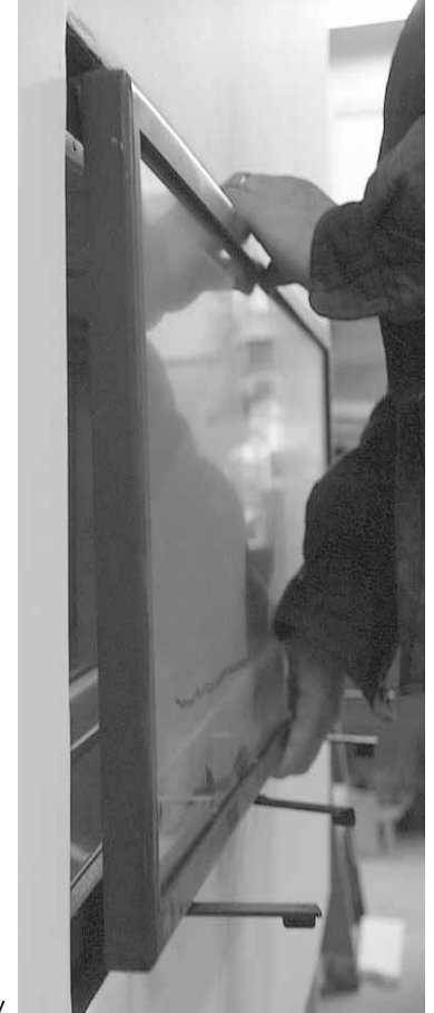
Figure 22 - The Vertical Installation of the Glass Panel Assembly
